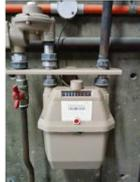
Newer buildings may also contain an MDL. These are remote reading units for all the meters (common area and apartments). The remote reading units send the gas usage on a weekly basis to the gas companies. It looks like this:
